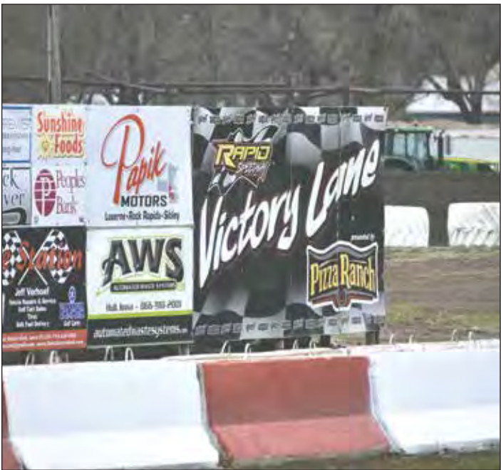
The new signage in the pit area has been rebuilt after last year's flooding at Rapid Speedway (above). The view of Rapid Speedway down the front stretch with a brand new fence around the outside of Turns 1 and 2 that was destroyed by flooding in June of 2024 (below).
